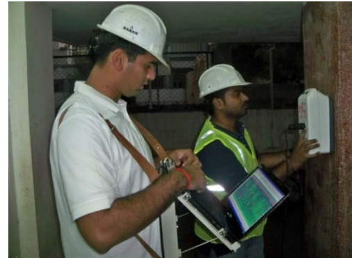
GPR Survey in progress
