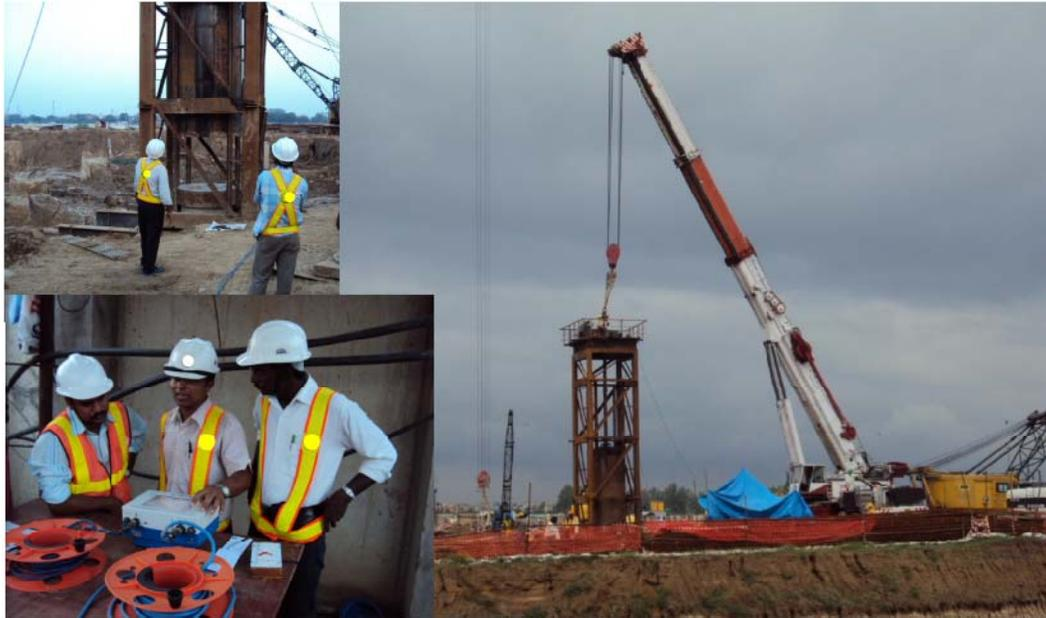
Figure 3 HSDPT in progress using 35ton hammer
