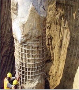
Figure 8 Picture of Defect post LSIT and Excavation
