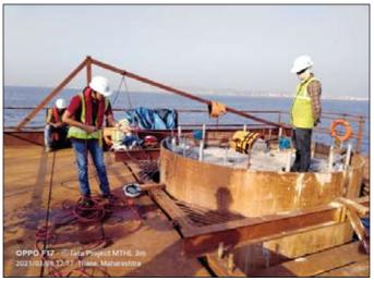
(a) CSL Test in Progress on 3m pile
