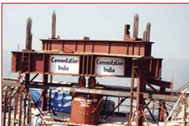
Fig. 2: Load test using anchor piles
