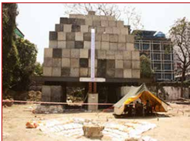
Fig.1: Load test using kentledge arrangement
