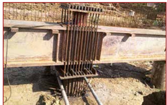
Fig. 4: Pull-out arrangement on a working pile at Kalma
