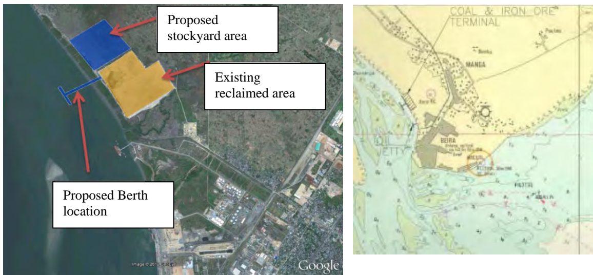
Figure 1: The proposed site location of stock yard and berth location at Beira, Mozambique
