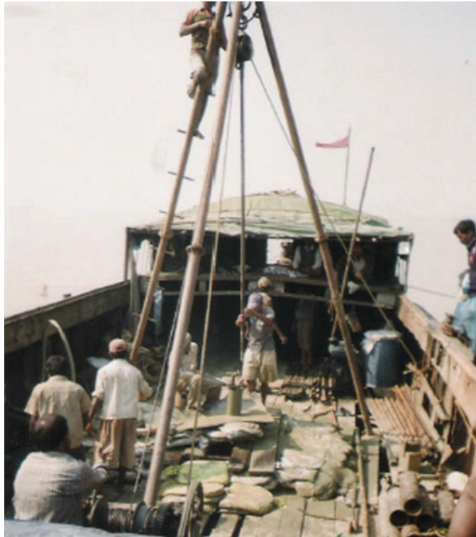
Fig. 2 Subsurface exploration in progress
