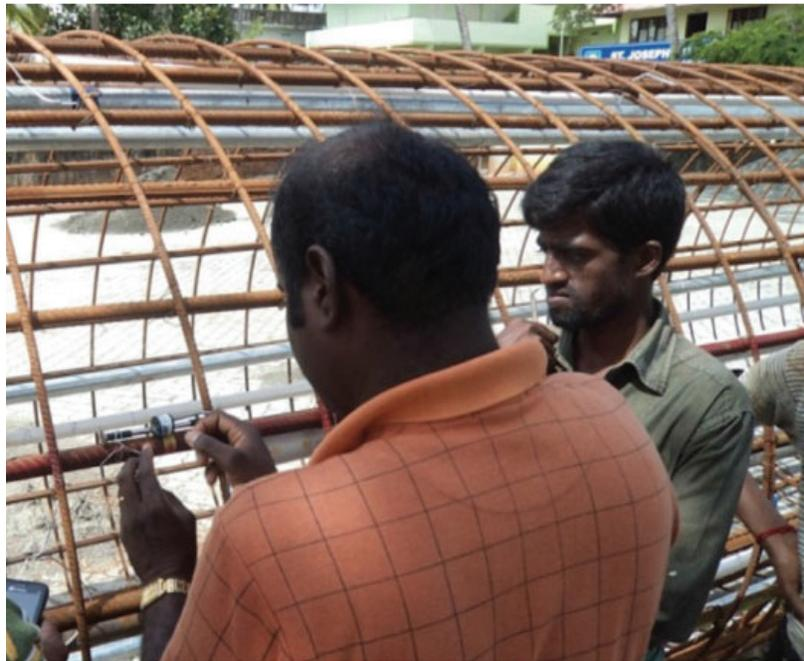
**Fig. 1** Strain gage installation in progress
