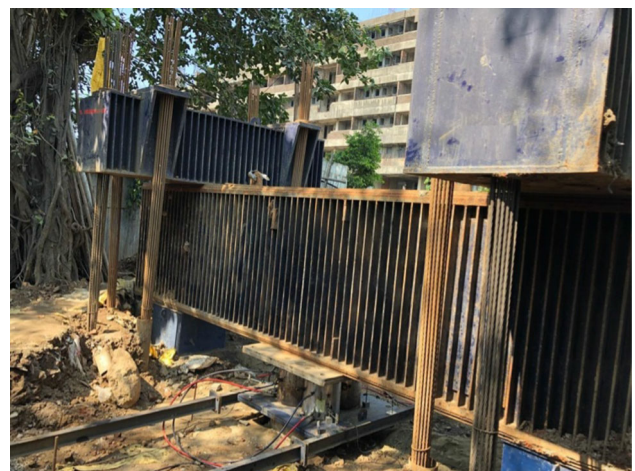
Fig. 5 Vertical load test in progress with 12 rock anchors
