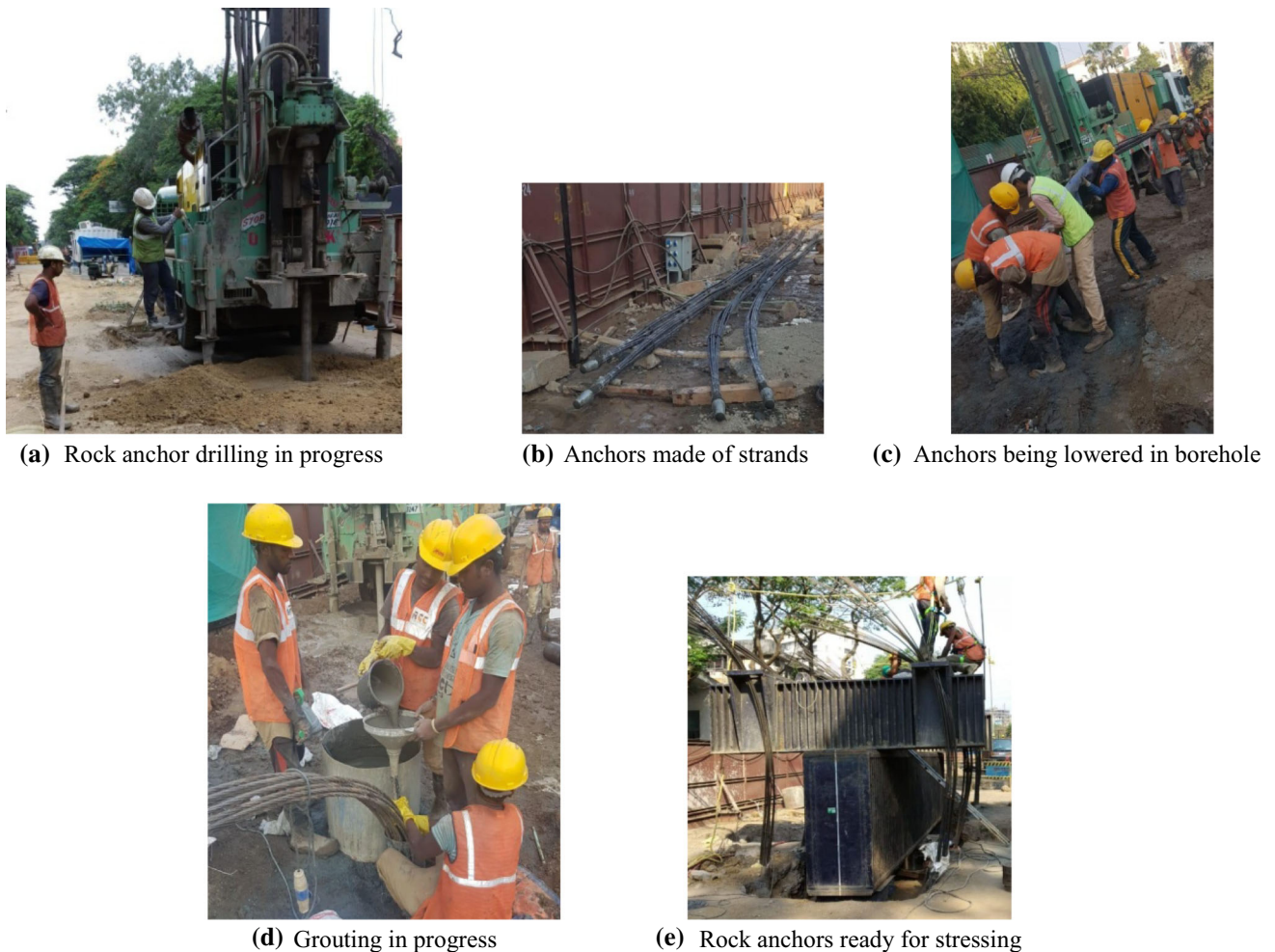
Fig. 1 Rock anchor installation procedure
