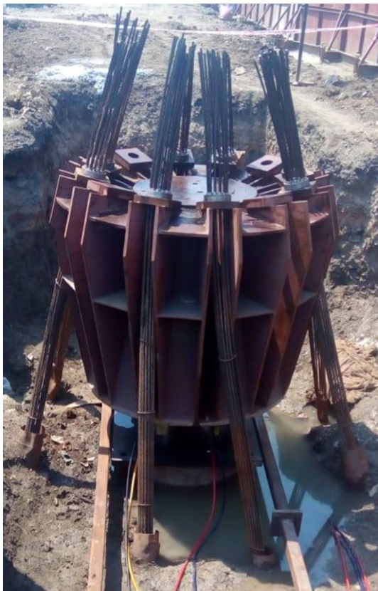
Fig. 4 Vertical load test in progress with crown girder setup
