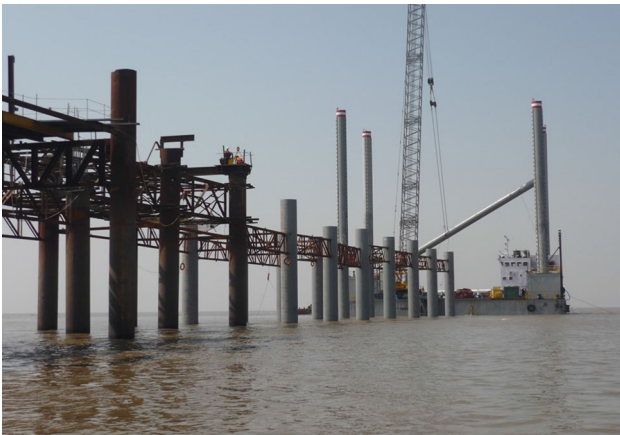
Fig. 9 A view of the partially completed Jetty
