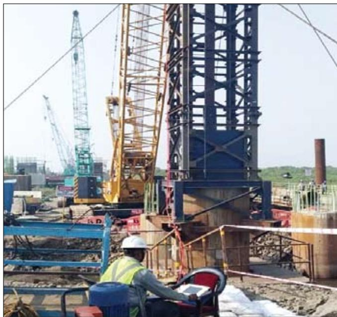
Figure 4 : High Strain Dynamic Pile Test in progress
