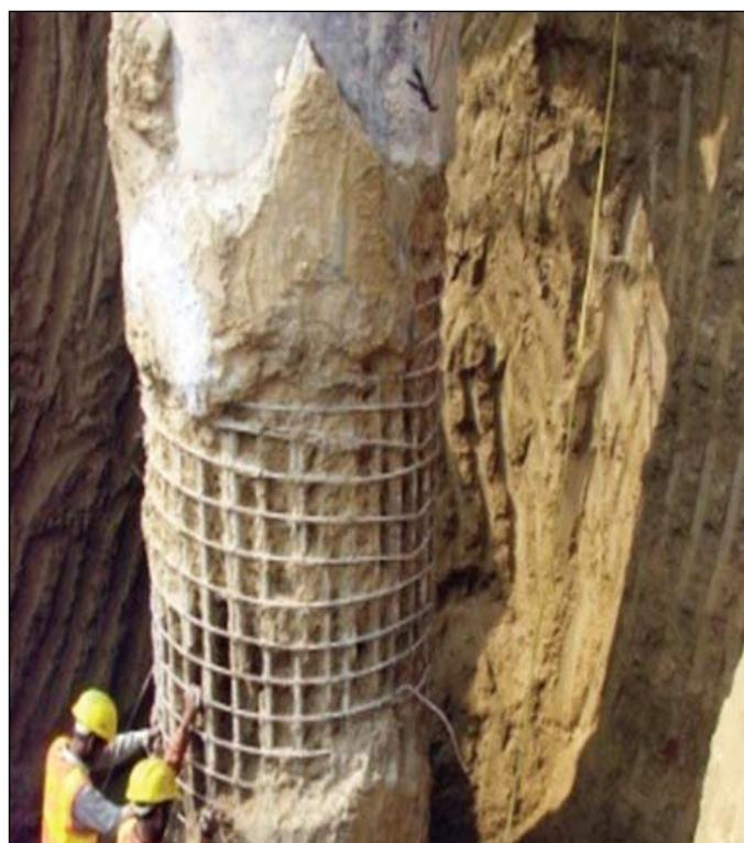
Figure 8 Picture of Defect post LSIT and Excavation
