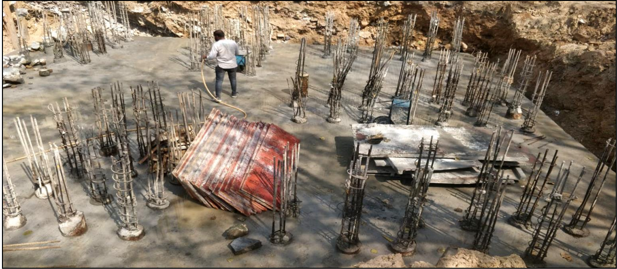
Figure 9 Picture of Closely Spaced Micro Piles
