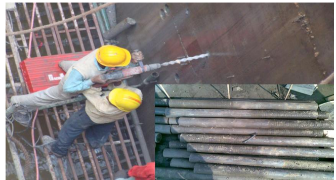
Figure 4. Drilling for Extra reinforcement along with anchor rods
