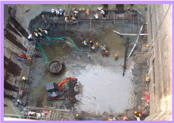
Figure 6. view after dewatering operation.
