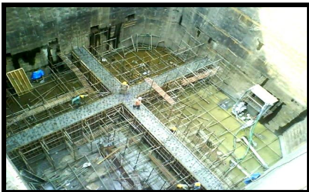
Figure 7. Finished bottom raft with beams.
