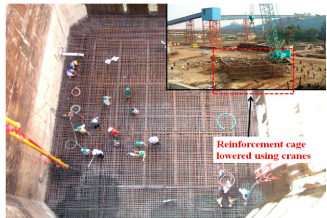
Figure 5. Reinforcements lowered for compartment 1
