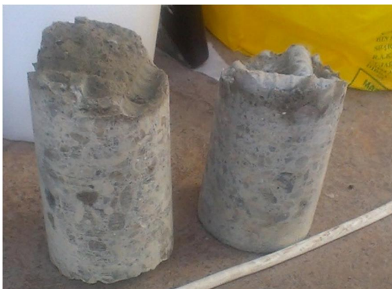
Fig. 5. Concrete core encountering main reinforcements. .
