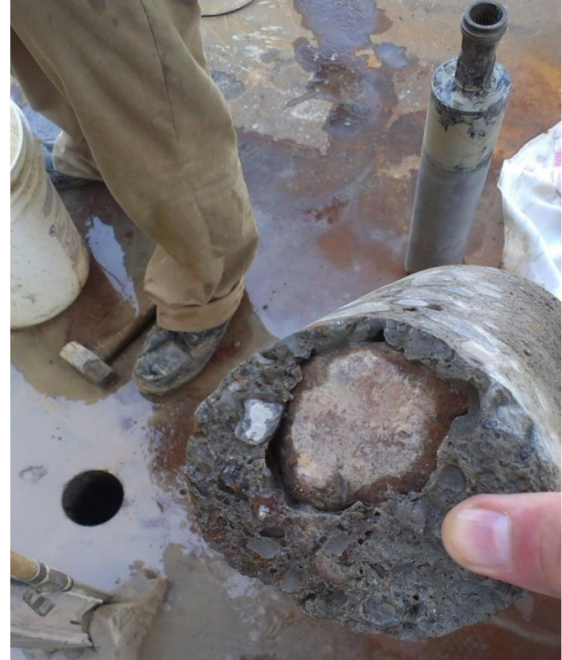
Fig. 9 Surprises in concrete cores
