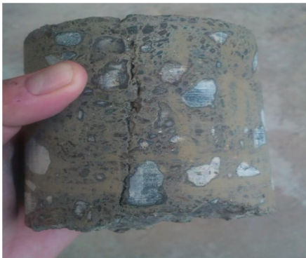
Fig. 8. Typical cracks observed in the top portion of the concrete core.
