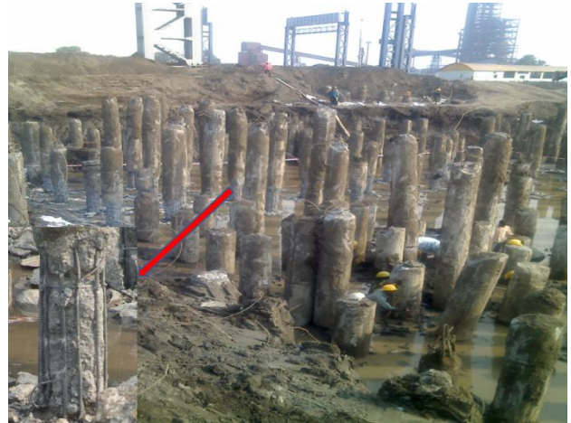
Fig. 4 Excavated area for checking pile profile
